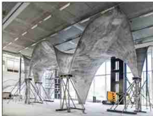
Fig 1 Ultra-thin curved roof using novel formwork system
